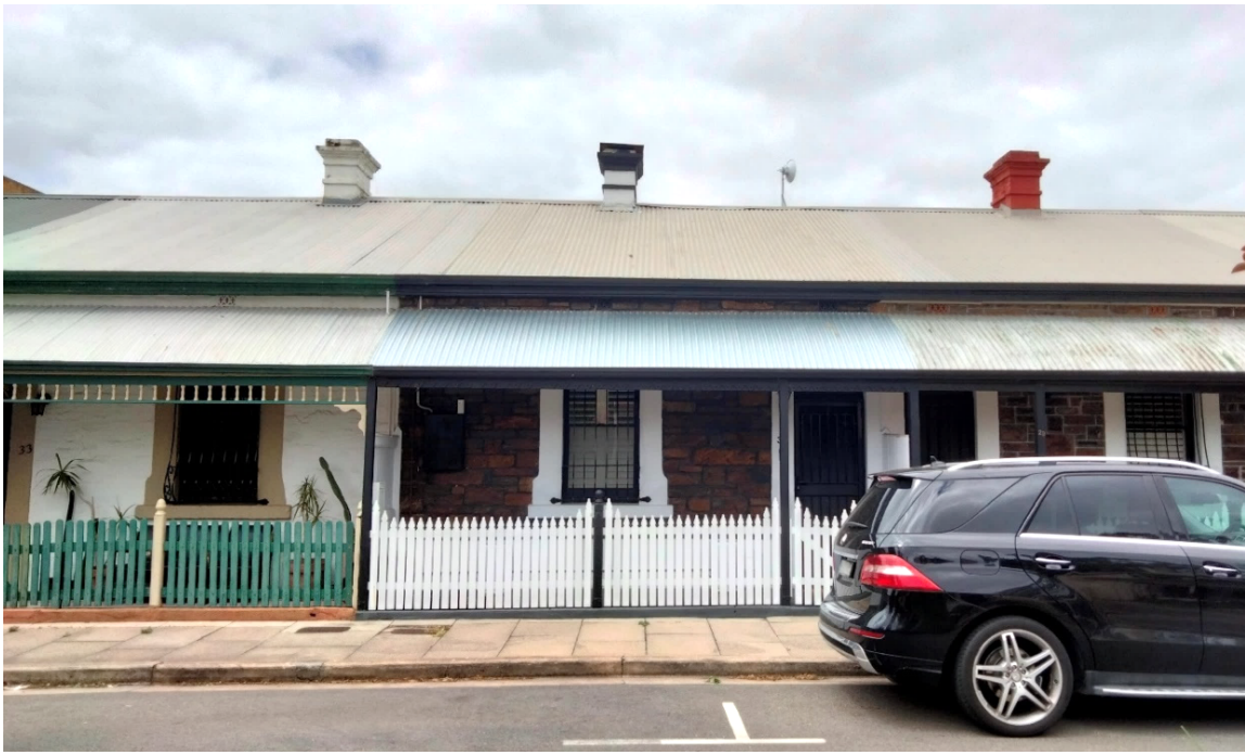
Photo 3.1 - Subject site viewed from McLaren Street
